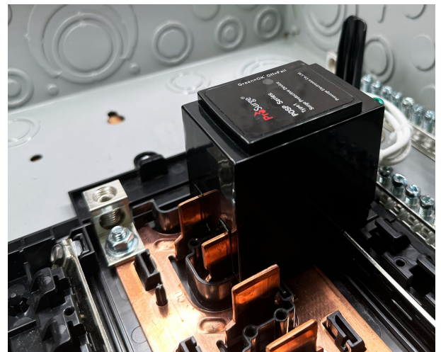
Fig. 1. Plug- on install on Load center
